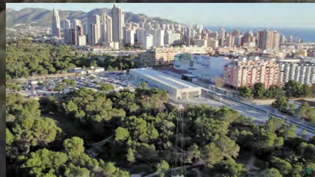
Red Tram D'Alacant in Benidorm, one of the points where FCC Construcción's Digital Railway Infrastructures project is being applied.
