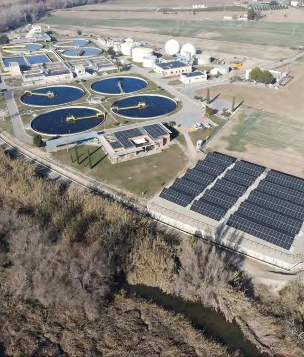
Wastewater Treatment Plant (WWTP) of Lleida.
